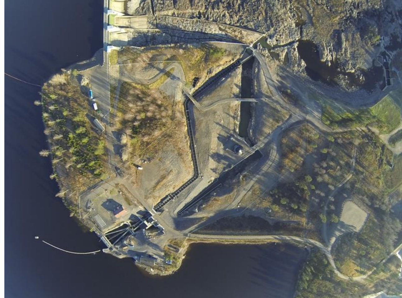
Fish ladder at the Stornorrfors powerplant in the Ume river.
