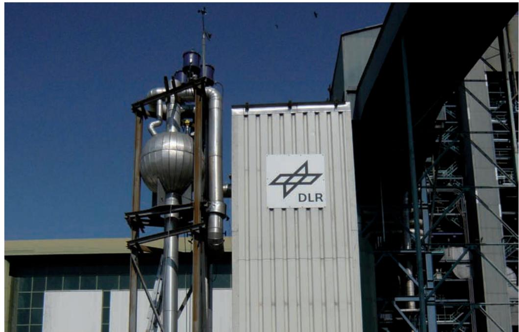
Figure 17: Latent storage system with 700 kW power, 1h storage capacity, Source: DLR.
